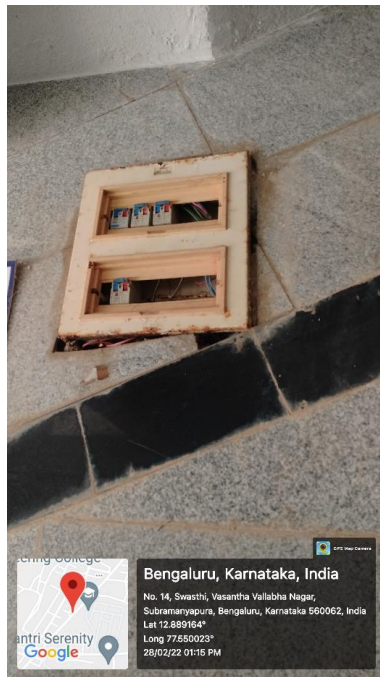
Figure 5-5: Load distribution box MCBs at each floor
