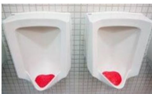
Figure 4-26: Waterless urinals
