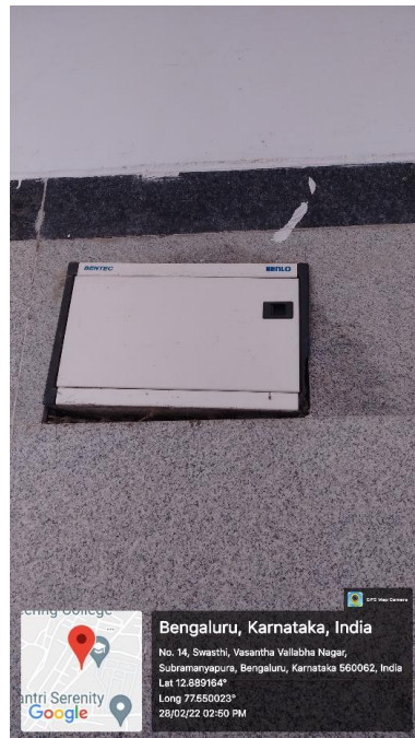
Figure 5-5: Load distribution box MCBs at each floor
