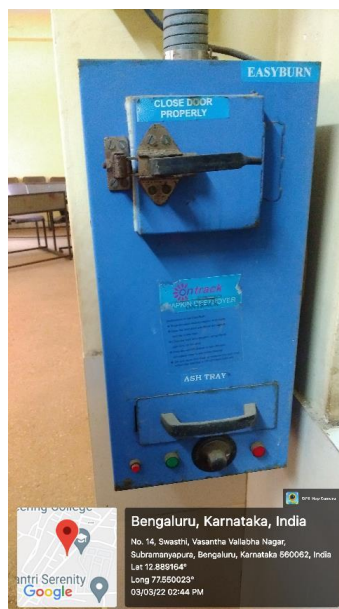
Figure 6-5: Bio – waste management - Napkin incinerator
