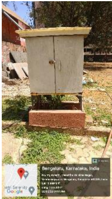
Figure 5-4: Sub -distribution panels for CS/IS block
