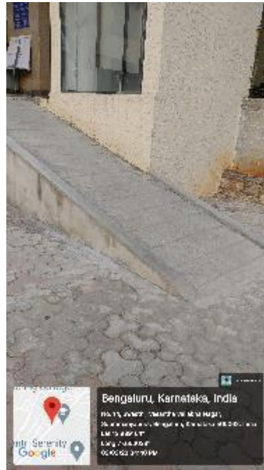
Figure 8-4: Ramp facility at Dr. Sir. M. Visveswaraya block
