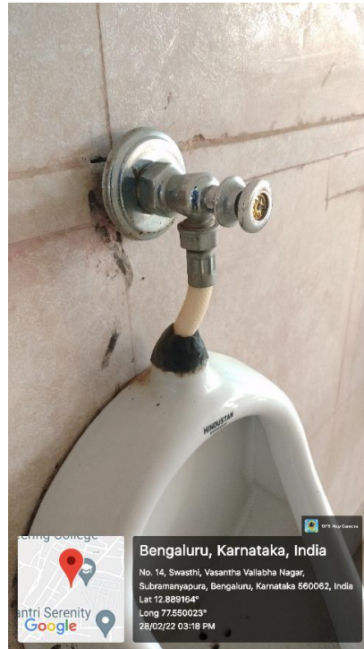
Figure 4-20: Push type tap for urinals
