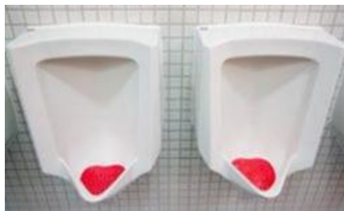
Figure 4-28: Waterless urinals
