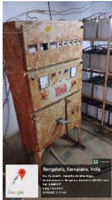
Figure 5-4: Sub -distribution panels for CS/IS block
