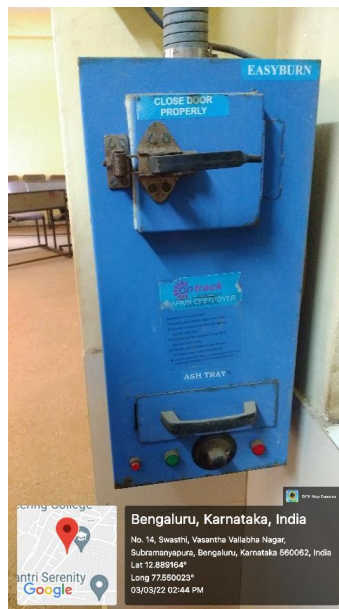
Figure 6-5: Bio – waste management - Napkin incinerator
