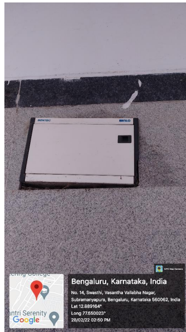
Figure 5-5: Load distribution box MCBs at each floor
