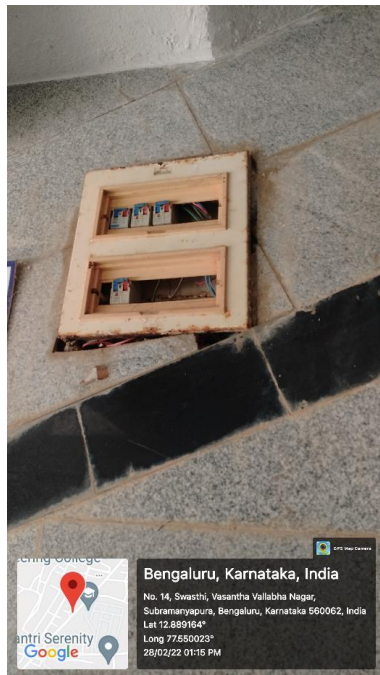
Figure 5-5: Load distribution box MCBs at each floor
