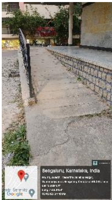
Figure 8-5: Ramp facility at Dr. A.P.J. Abdul Kalam block
