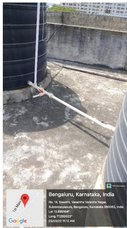
Figure 4-9: Interconnection between tanks with valve control
